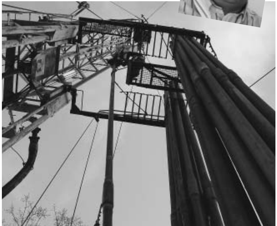
The Basle deep-drilling rig
